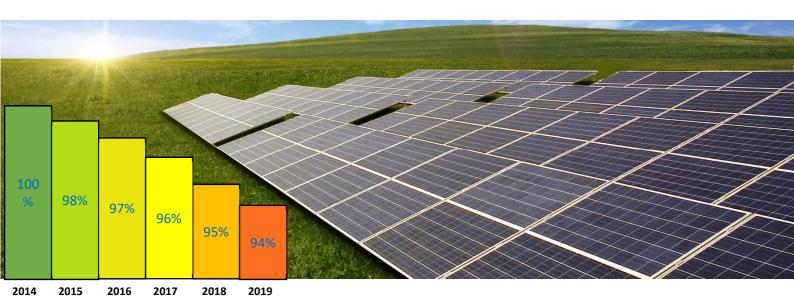
Photovoltaic systems are affected by decreasing yields already in the first few days - weeks of operation. This yield reduction occurs due to the light-induced degradation (LID) in photovoltaic modules.
